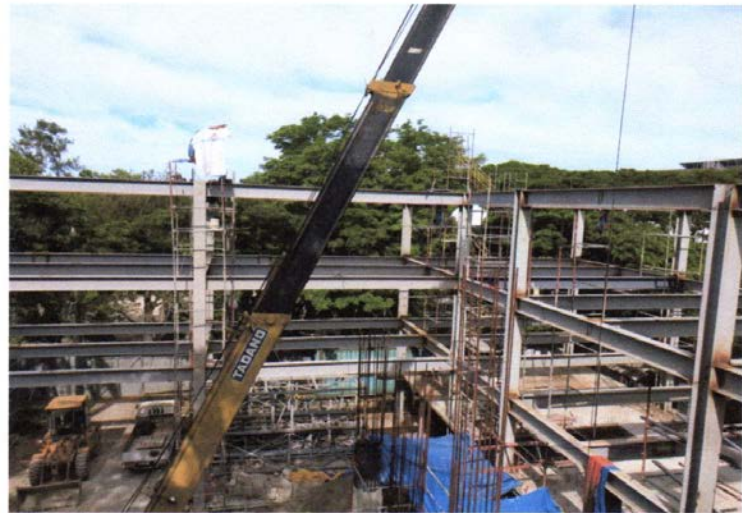
INSTALLATION OF WIDE FLANGE STEEL BEAMS AT CENTRAL & EAST WINGS
