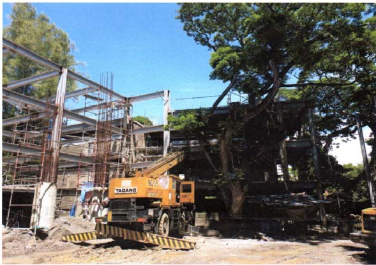
STEEL BEAM WIDE FLANGE INSTALLATION & FULLWELD OF CONNECTIONS
